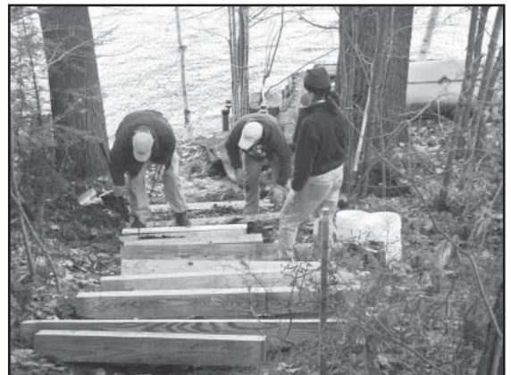
Infiltration steps help to capture and infiltrate stormwater runoff, preventing nutrient filled runoff from entering the lake.
