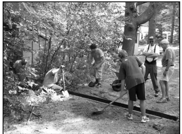
Raymond Pond - Volunteers Install Rubber Blade Diverter to Direct Water into Vegetation.
