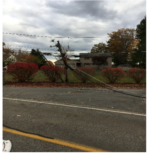
Power pole/lines blocking road
