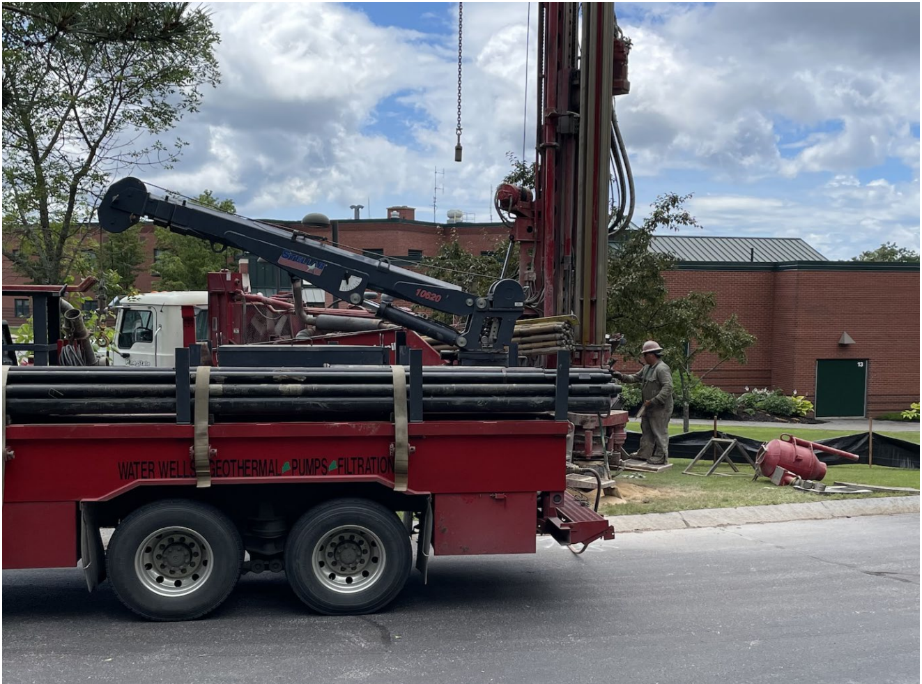
Well drilling at Raymond Elementary School
